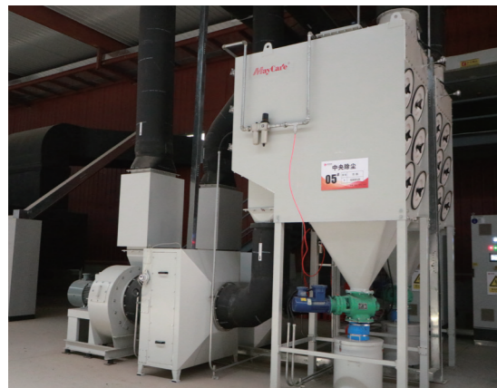
CARTRIDGE DUST COLLECTOR Applied in automotive components
