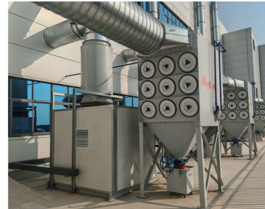
CARTRIDGE DUST COLLECTOR Applied in automotive sandblasting, grinding, and welding dust control
