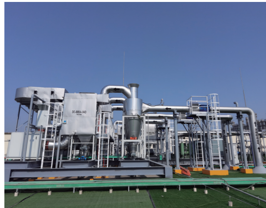
CARTRIDGE DUST COLLECTOR Applied in the treatment of explosive dust in photovoltaic polycrystalline silicon
