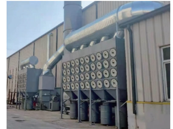
CARTRIDGE DUST COLLECTOR Applied in welding processes
