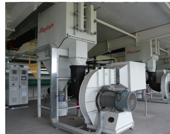
CARTRIDGE DUST COLLECTOR Applied in lithium battery cell production lines
